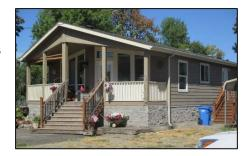
The end result is an open foundation or a higher crawlspace that allows floodwaters to flow under the first floor. Most <u>grant programs</u> that fund relocation can also help fund elevation projects. Raising the lowest floor above the base flood elevation can also lower flood insurance premiums by up to 80%.
