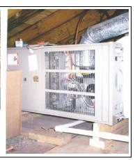
A flood in this house's crawl space resulted in over \$4,000 in damage to ductwork alone. The owner elevated the air conditioning compressor and relocated the furnace and ductwork into the attic. The result is an empty crawl space, no longer subject to floodwater damage.
