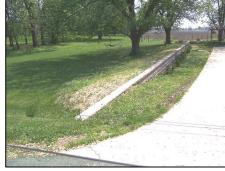
Do not backfill against your crawlspace wall because that may block the openings (see the next section). Also, if your crawlspace floor ends up below the fill level on all sides, it could result in higher flood insurance premiums.
