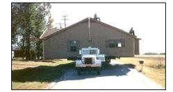
b. Elevate: If you don't have a high velocity flood hazard and you will receive a warning, the next safest alternative is to (3) elevate the building above the expected flood level. Buildings with crawlspaces in low velocity areas are the easiest to elevate. The steps are explained in a brochure from the International Association of Structural Movers and in FEMA's guide, Above the Flood: Elevating Your Flood-Prone House (P-347).
