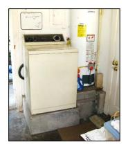
g. **Elevate your utilities:** Heating, air conditioning and electricity are vital utilities to make a building livable. If they are knocked out, it will delay repairing, rebuilding and reoccupying. One way to protect these utilities is to elevate them above the flood level, as in the example, below. Don't forget to elevate electrical outlets, too.
